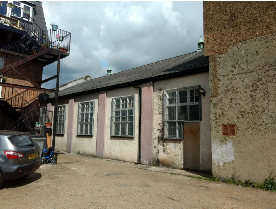
South facing elevation facing Herga Mansions
